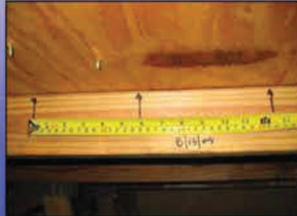
Fastener Spacing
